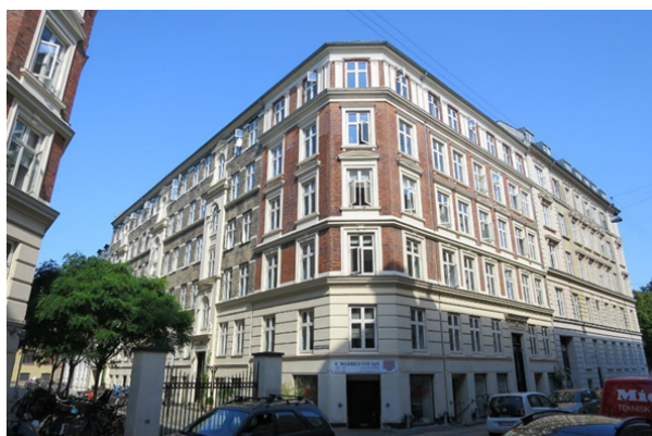
Fig. 1. Case study building.
